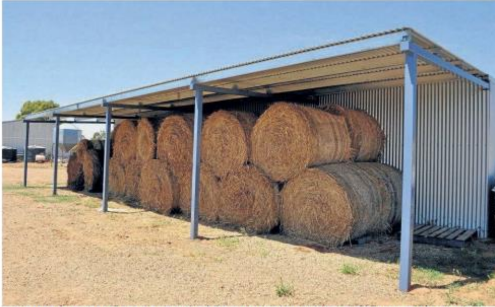
This recently completed hay shed was built by several inmates who are skilled welders and builders. This is an example of the way the centre is able to utilise their talents.
