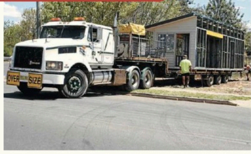
THEN: February 12, 2013 The house is moved into place.
